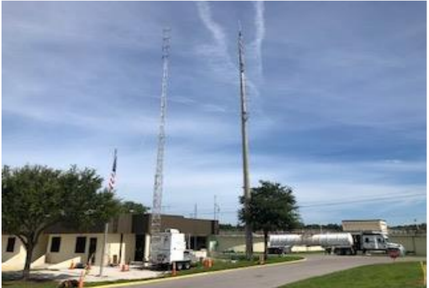
Figure 2. Radio Communications Tower 2
