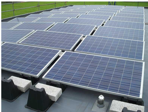
Fig. 11: Ballasted Flat Roof Mounted Solar System (Gupta, 2018)
