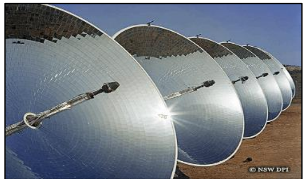
Fig. 24: A Parabolic Solar Dish is a mirrored shape like a satellite antenna. It concentrates light energy on a receiver. - Solar power at White Cliffs (Dpi, 2009)
