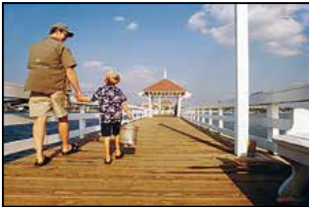
Bridge Street Pier
