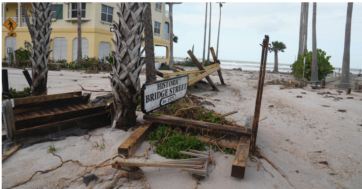
Figure 12 – Hurricane Helene Damage on Anna Marie Island
