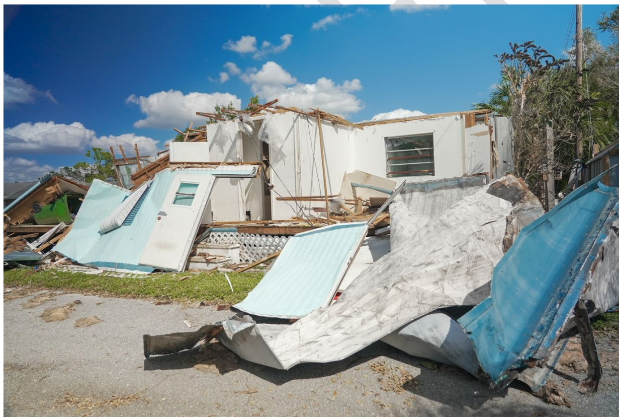
Figure 11 – Hurricane Milton Modular Home Damage
