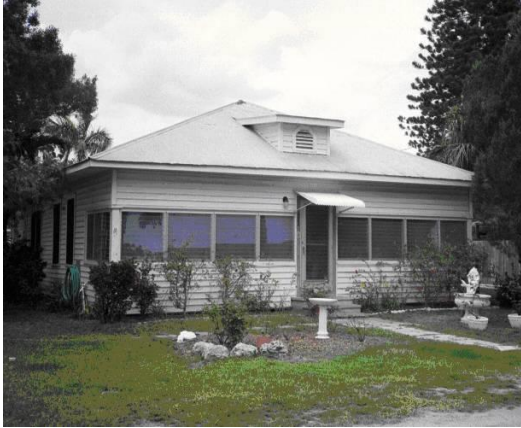
Figure 9 - 65: Frame Vernacular Style - pyramidal roof
