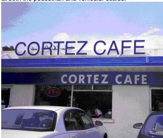
Upper sign band too large for facade, lower band is better
