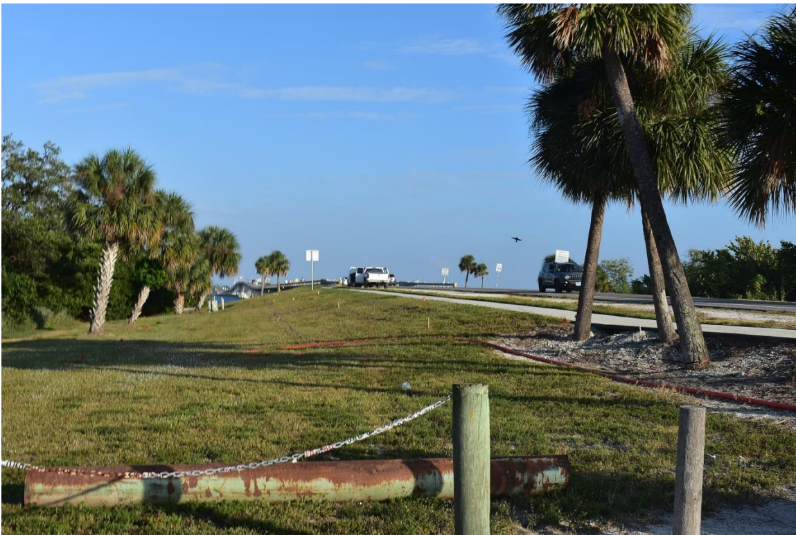
STREET VIEW TOWARD BRIDGE APPROACH
