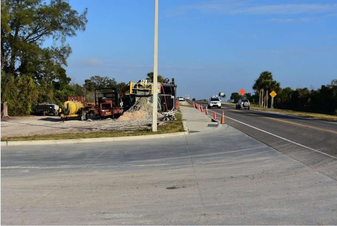
VIEW EAST ALONG SUBJECT SITE (EAST END OF SUBJECT SITE)
