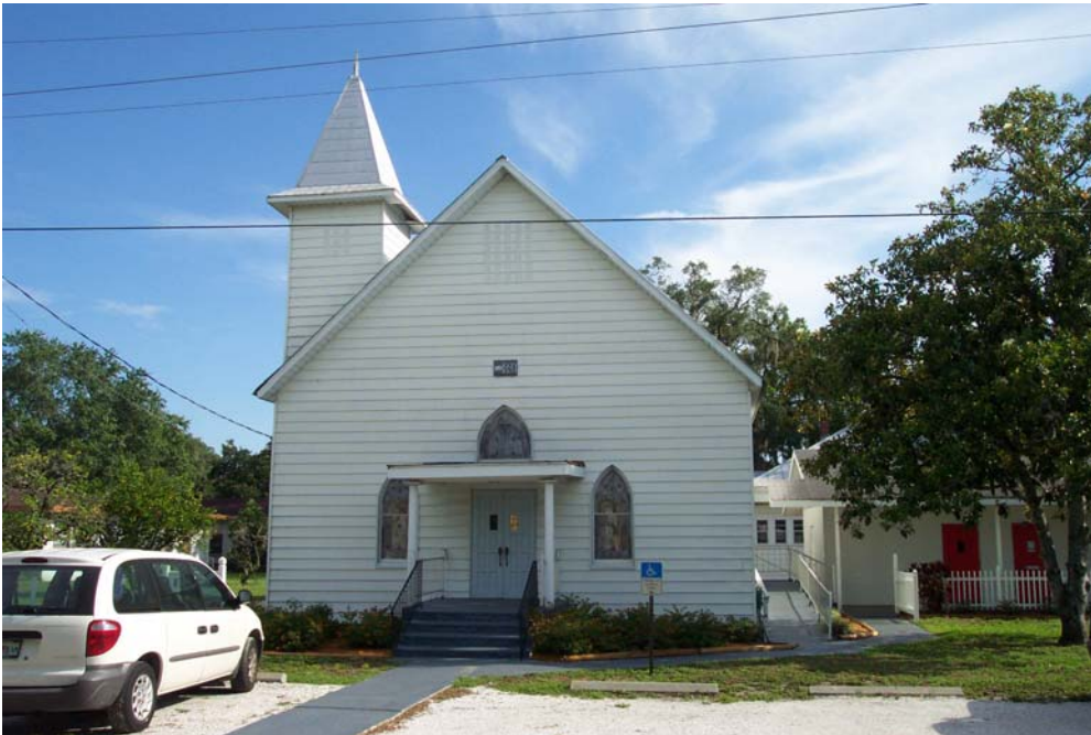
Figure 5.10 MA00766-Parrish United Methodist Church-12140 69th St. E. - Current Photograph Renker Eich Parks Architects
