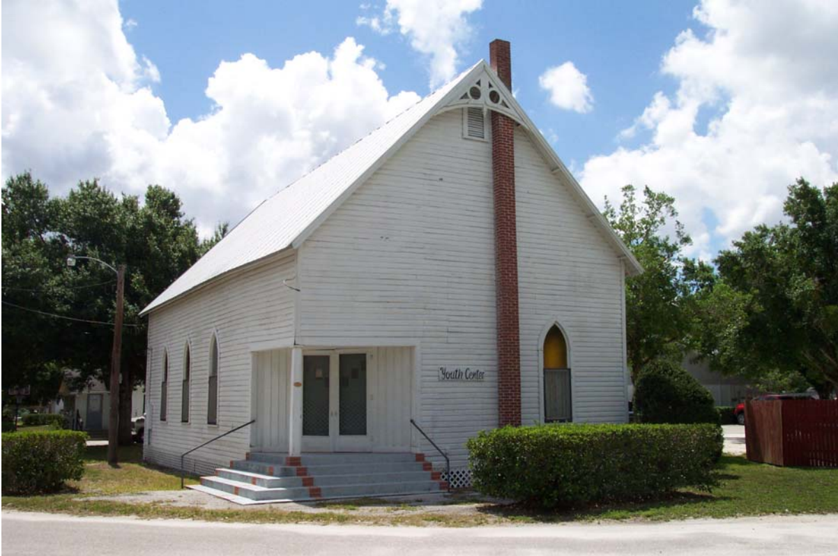
Figure 5.21 MA01566-First Baptist Church Youth Center-6918 121st Ave. E. - Current Photograph
